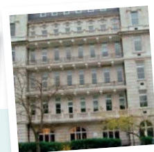
Royal London Hospital for Integrated Medicine (formerly the Royal London Homoeopathic Hospital)
